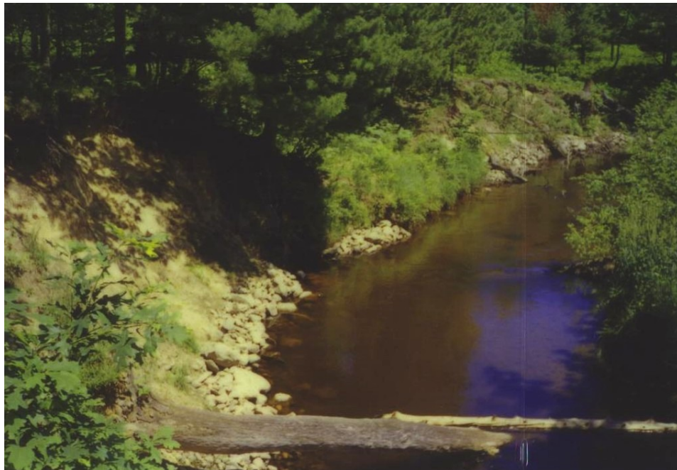
Figures 3.12. and 3.13. Streambank stabilization at Cedar Creek before (top) and after (bottom) using a combination of traditional and soft treatments.
