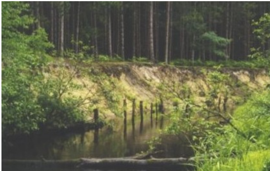
Figures 3.14. An eroding Streambank on Winnepesaug Creek prior to receiving bioengineering (soft) stabilization treatments.
