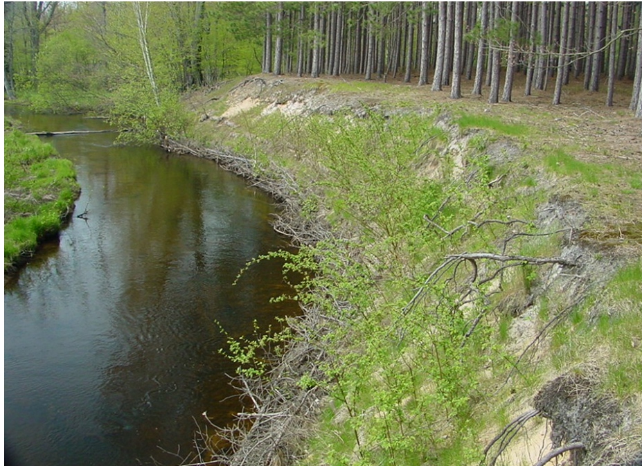
Figures 3.15. Winnepesaug Creek stream bank after receiving bioengineering (soft) treatments. Note the native vegetation which has established on the upper slope.
