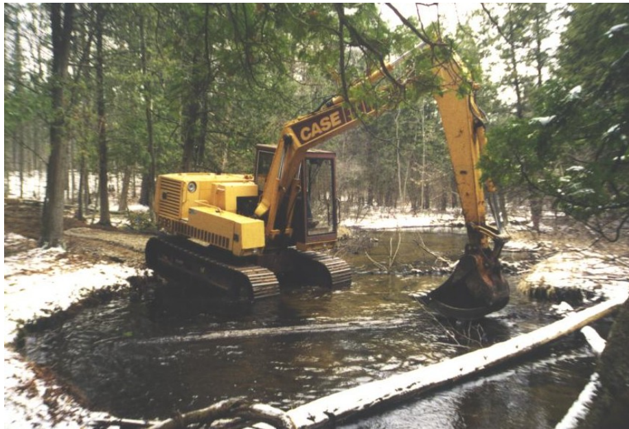
Figures 3.3 and 3.4. Construction of Big South Branch Pere Marquette Station 1 (MS-GB-1)(top) and Tank Creek (T-GB-1)(bottom) gravel bars.
