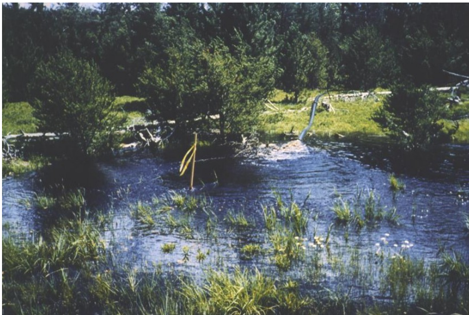
Figures 3.6 and 3.7. The Stream Sweeper TM dredges sand (top) and pumps sediments approximately 800 feet to an upland site (bottom).
