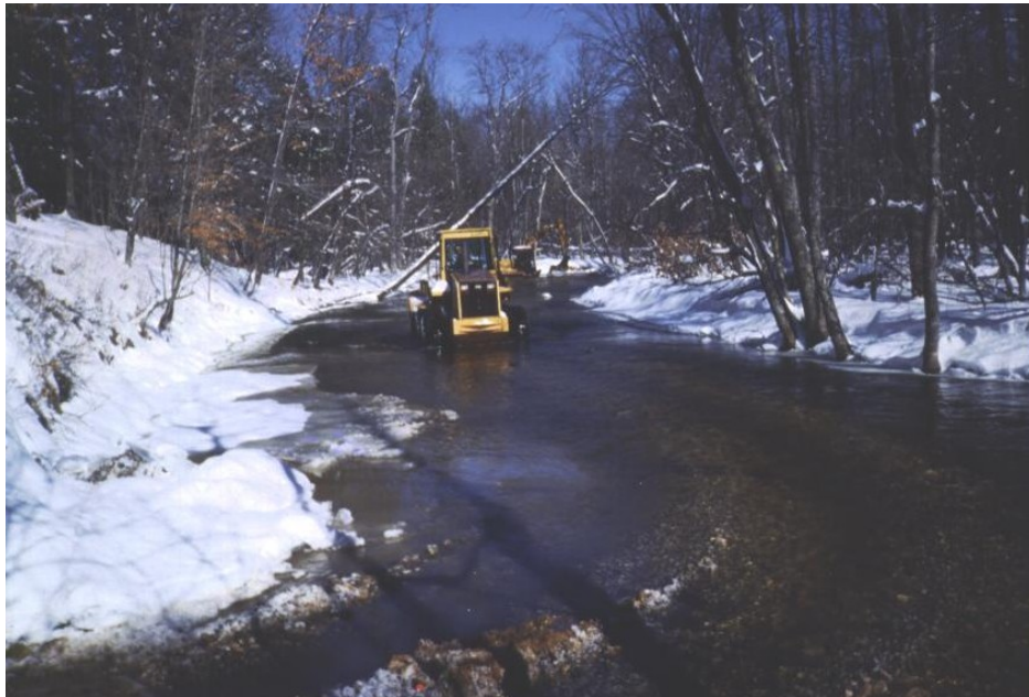
Figure 3.5. Placement of gravel during construction of Big South Branch Pere Marquette Station 2 (MS-GB-2) gravel bar.
